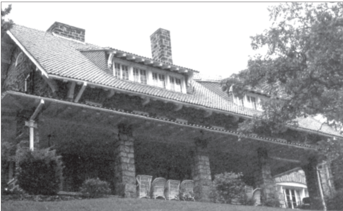
“Pulpit Rock,” Little Sewickley Creek Road, Edgeworth. Built for Samuel C. Walker. Rutan & Russell, architects, 1901
